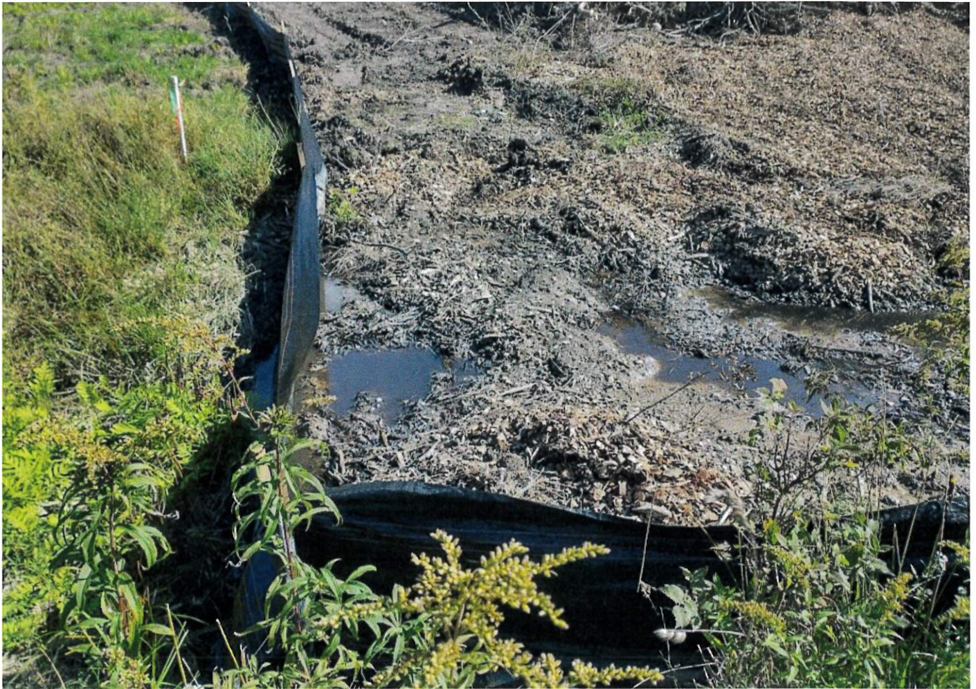
Fill within Wetland up to Silt Fence
