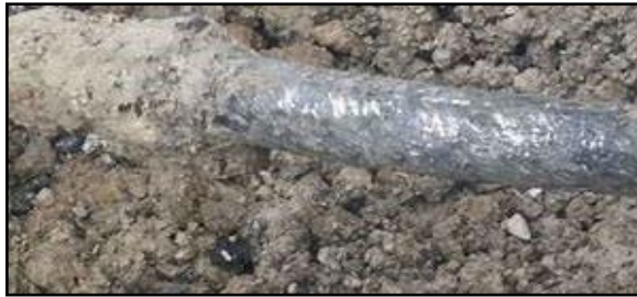
Lead: The pipe will appear dull and soft but will turn a shiny silver color when scratched. A magnet won't stick.
