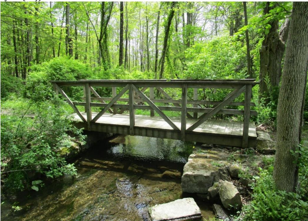
Figure 1.16 A contemporary pressure treated wood bridge has replaced the historic wood deck bridge with rustic cedar log railings. Built atop the historic stone footings, the new bridge is sized to accommodate pedestrians rather than vehicles. It serves as the primary access to the Madison Lewis Woodland trails from Robin Brae Drive. (MLW-Bridge 2017 May 10 (40))
