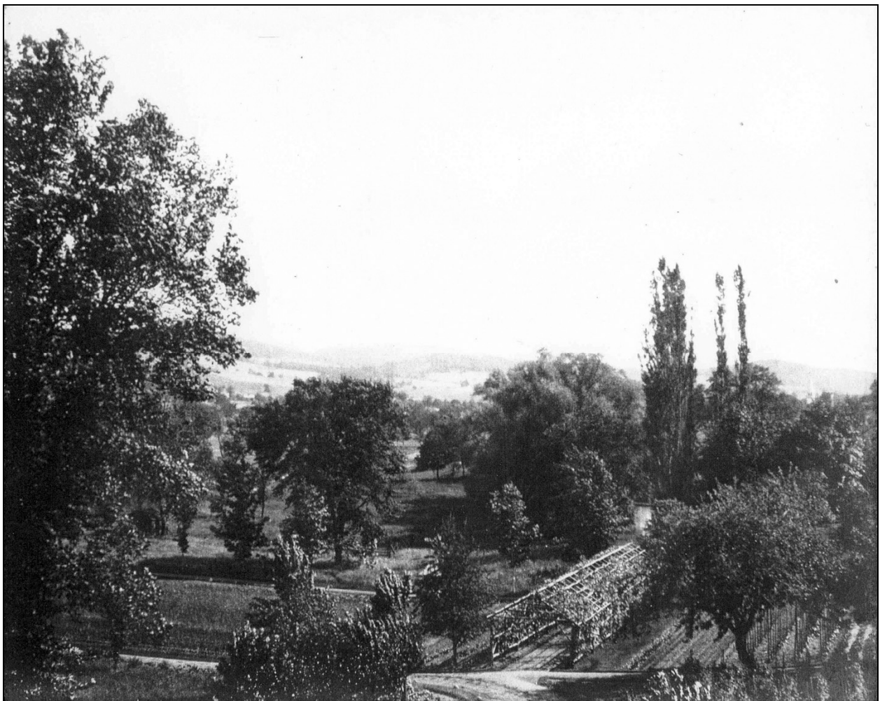
Figure II.28. View looking south from the carriage house and stables show a drive curving downhill, past the orchard to the right and an arbor, center. The drive continues to the left to the woodlands. The arbor-covered secondary drive runs parallel to the orchard and leads to the constructed pond, visible at end of the drive. Courtesy Warwick Historical Society. (R-MLW-VW-BA-FromStable-1902.jpg)
