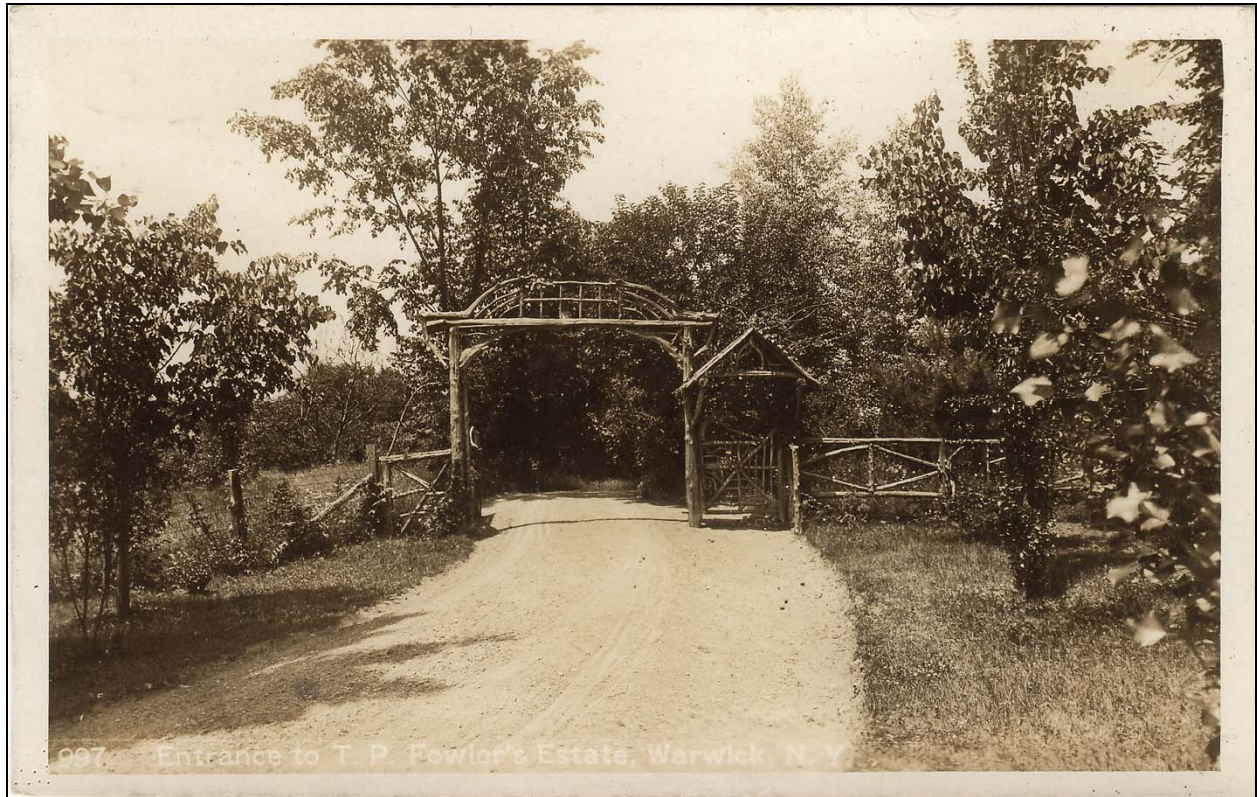
Figure II.17. View along the curving drive shows the rustic pole and twig gate shown in the previous image and additional features at the entrance into the estate. A pedestrian gate is located to the side of the carriage gate. A simple roof provides shade, and wooden fence extends to either side of the gate. To the left, the fence connects with a wooden post and wire fence that restricts access onto the estate grounds. Deciduous trees of varying sizes line the drive with the woodlands visible beyond. Courtesy Steve Gross. (R-MLW-SG-GateDrive-1927-front.jpg)
