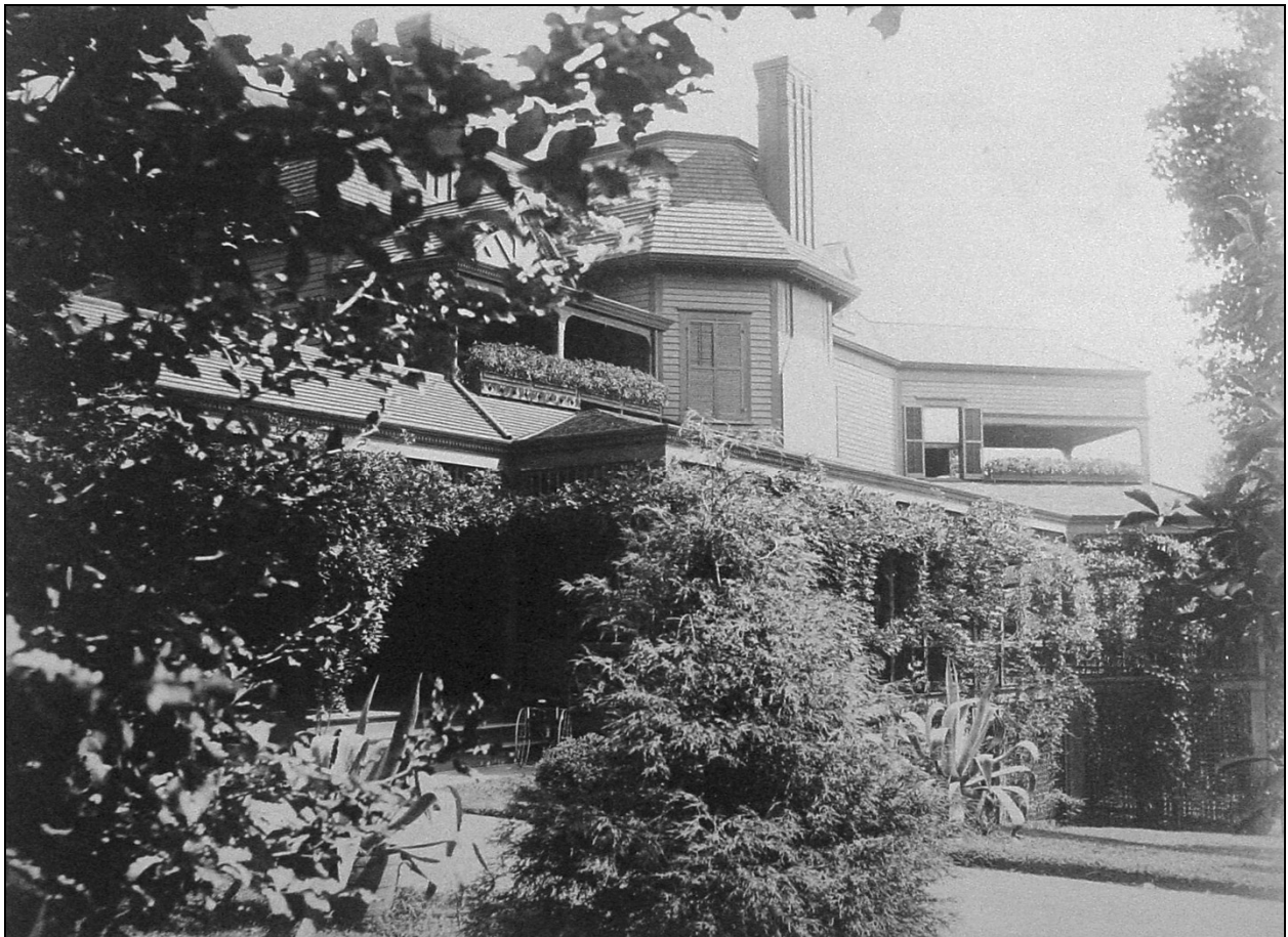
Figure II.23. This view looking toward the southwest corner of the Fowler mansion shows the plantings that flank the drive, climb on the porch and appoint the landscape near the building. The planting character is quite showy and is in a different style from that of the naturalistic character of the estate woodlands. Courtesy Steve Gross. (R-MLW-VW-BA2-HousePlantings-1905.jpg)
