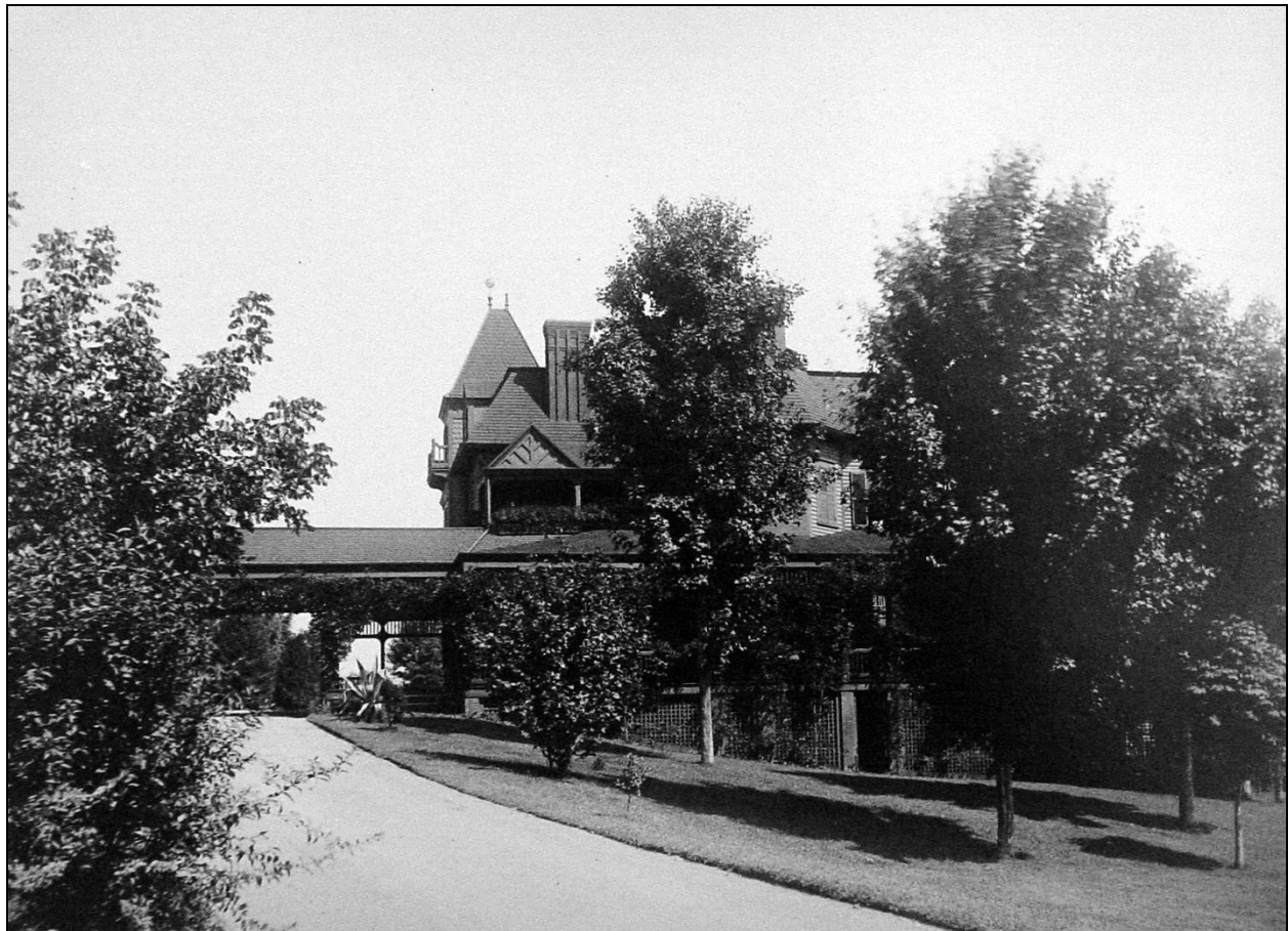
Figure II.30. View looking north along the Belair driveway shows the drive running under a porte-cochere that extends from the west façade of the house. A collection of trees is seen on the gently sloping hillside south of the house. Another tree is visible along the drive edge. Vines grow on the façade of the house and porte-cochere. Courtesy Steve Gross. (R-MLW-VW-BA2-HouseDrive-1905.jpg)
