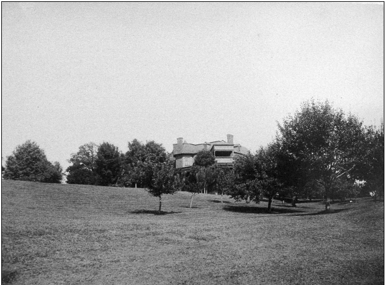
Figure II.11. View looking northwest shows a grassy slope with the Belair mansion and plantings beyond. Several young trees are planted in rows indicating that this may be the edge of the orchard to the southeast of the house. Courtesy Steve Gross. (R-MLW-VW-BA2-OrchardField-1900.jpg)
