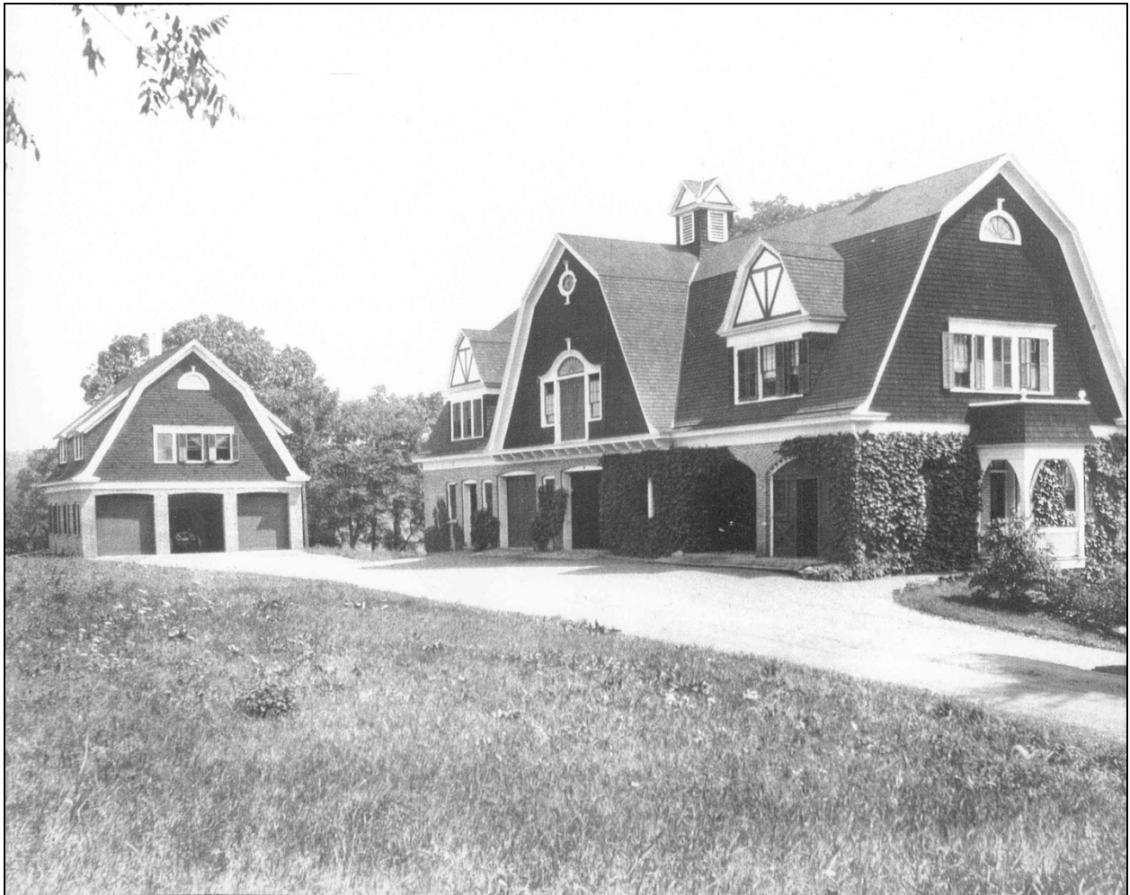
Figure II.24. This image looking northeast at the Fowler estate carriage house and garage shows a compacted gravel drive gently sloping away from the buildings. Rough turf covers the ground plane, while trimmed vines cover the first story of the stable. This carriage house was constructed in approximately the same location as the original carriage house. It appears that the carriage drive has been realigned and much of the earlier plantings have been removed. Courtesy Warwick Historical Society. (R-MLW-VW-BA-GarageStable-1910.jpg)
