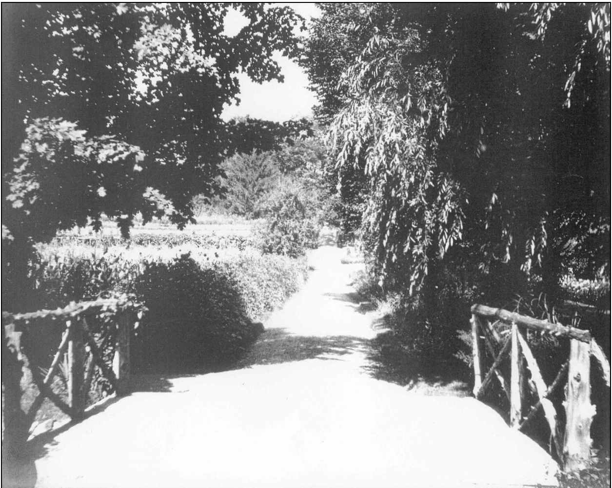
Figure II.14. This view along the carriage path shows a bridge edged by peeled cedar rails located near the edge of the woodlands. The rustic wooden bridge posts match the style of other landscape features. Mature deciduous trees overhang the end of the bridge while a flowering shrub row appears to edge the path with a corn crop behind it to the left. Courtesy Warwick Historical Society. (R-MLW-VW-BA-CarriagePath-1910.jpg)
